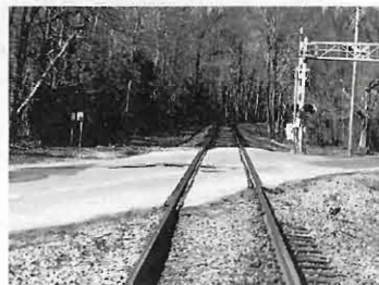
Left: Near Hughesville, the Chalk Point extension curves north and ties into the old Brandywine & Cedar Point RR at Gallant Green Road.
